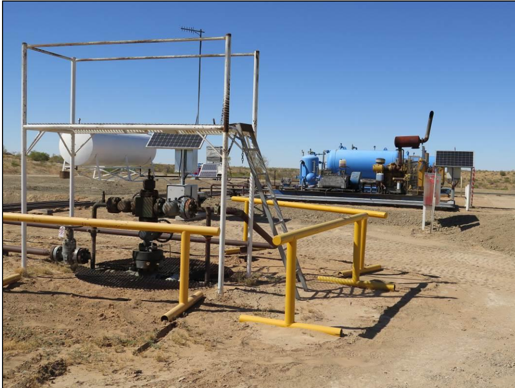
Plate 2: Jet pump, showing wellhead (foreground) and jet pump engine and fluid tanks (blue, in background)
